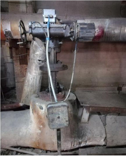
Fig. 5 The main feedwater control flow valve used in Nassiriyah thermal power plant.
