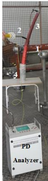
Fig. 5 Test setup consist of PD analyzer, HV circuit (1), PD sensor (2), cable termination (3) and oil tank (4).
