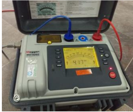
Fig. 10 Electric resistivity test of stress grading tubes.
