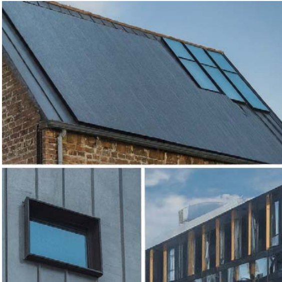
Fig. 3 Comparison of Opaque and Semi-Transparent BIPVT Systems
