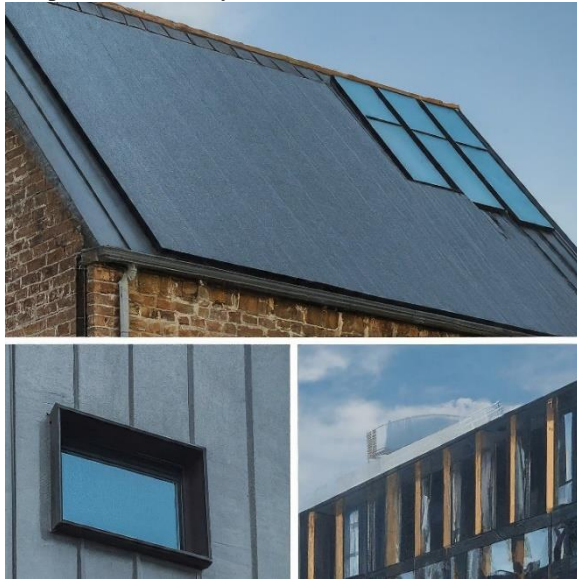
Fig. 3 Comparison of Opaque and Semi-Transparent BIPVT Systems
