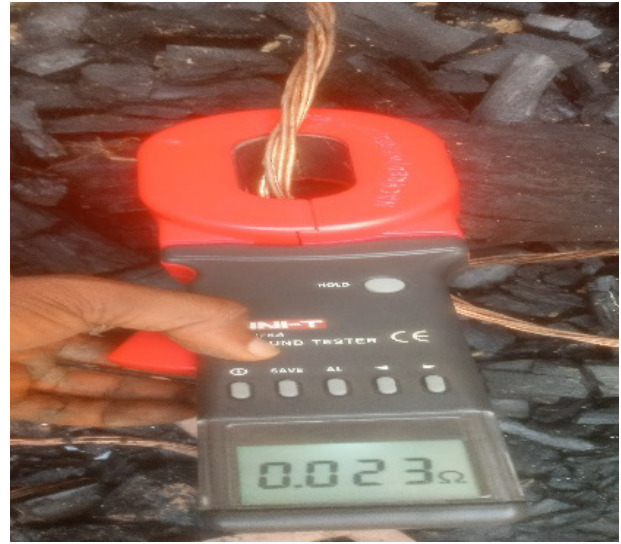
Fig 10. Ground Resistance Measurement Using UNI-T Ground Tester
