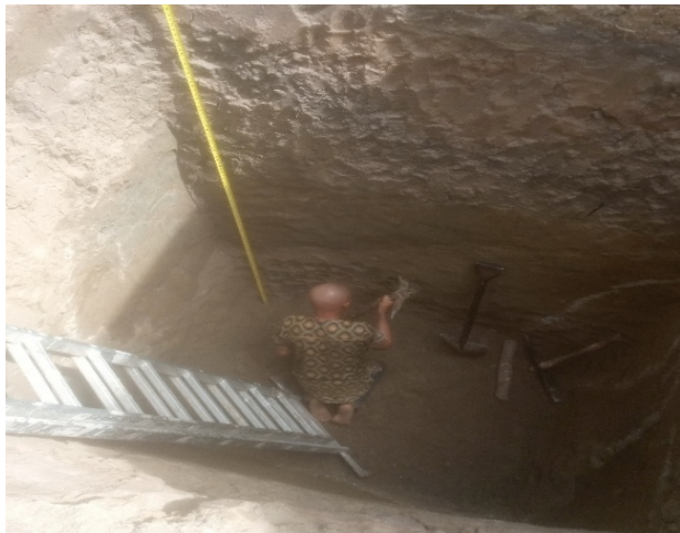
Excavation of a 3 m-deep pit ( 2.5\text{m} \times 2.1\text{m} ) at the site
