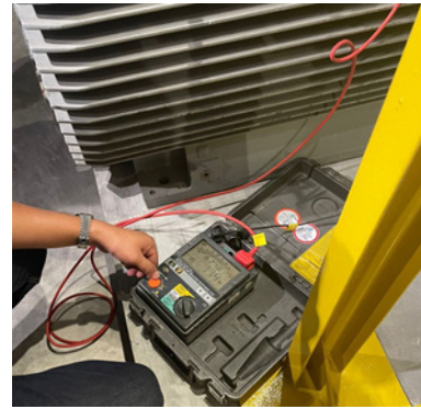
Fig 1. Insulation resistance testing
